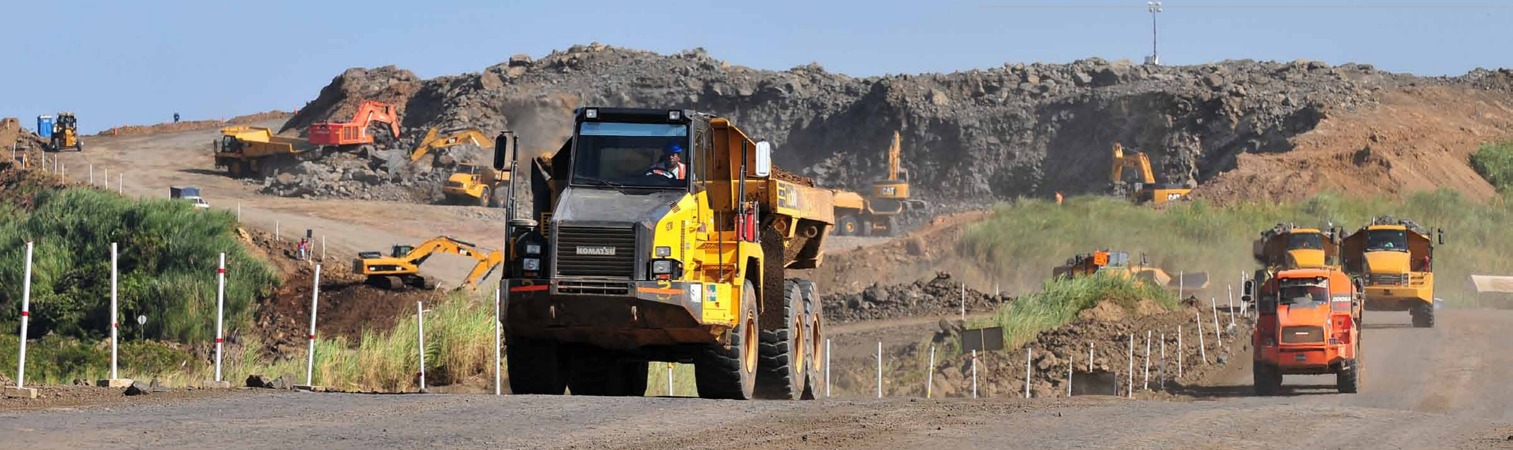
Excavation of access channel that connects the new Pacific Lock to the Culebra Cut
