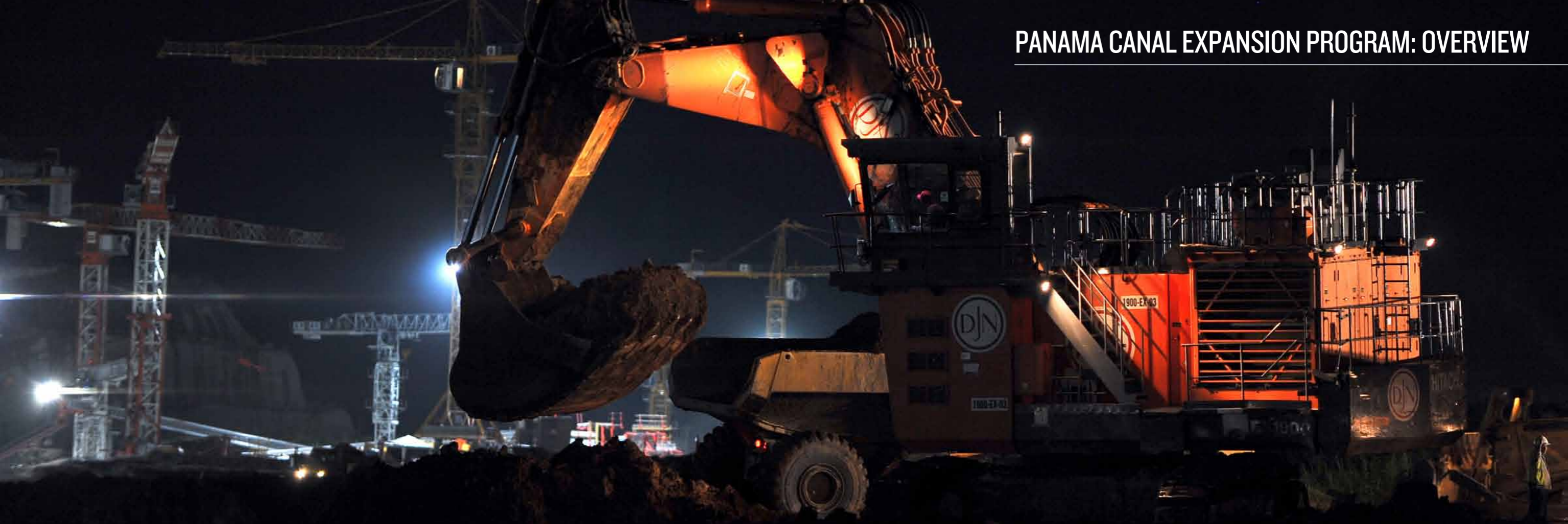
Construction continues day and night at the new Atlantic Lock site
