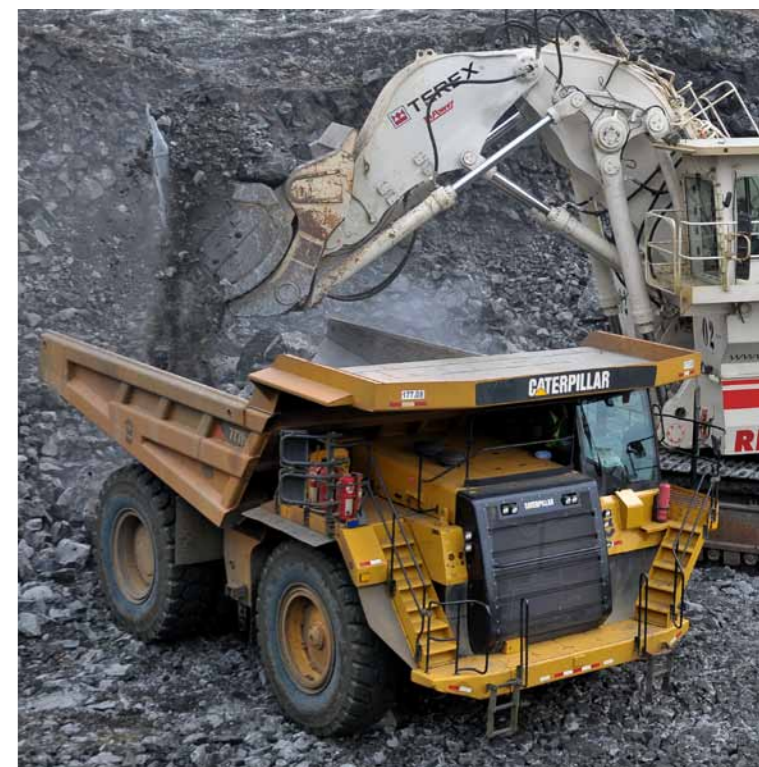
Basalt excavation of the access channel that will connect the new Pacific Lock to Gatun lake at Culebra Cut
