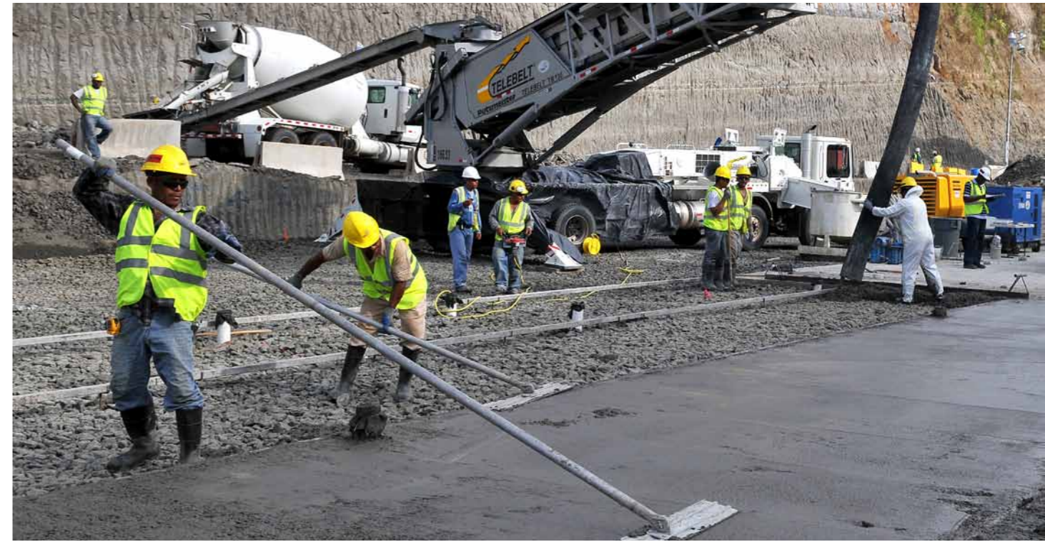
Leveling concrete base being placed so that forms and rebar can be installed effectively over it, and structural marine concrete can later be poured
