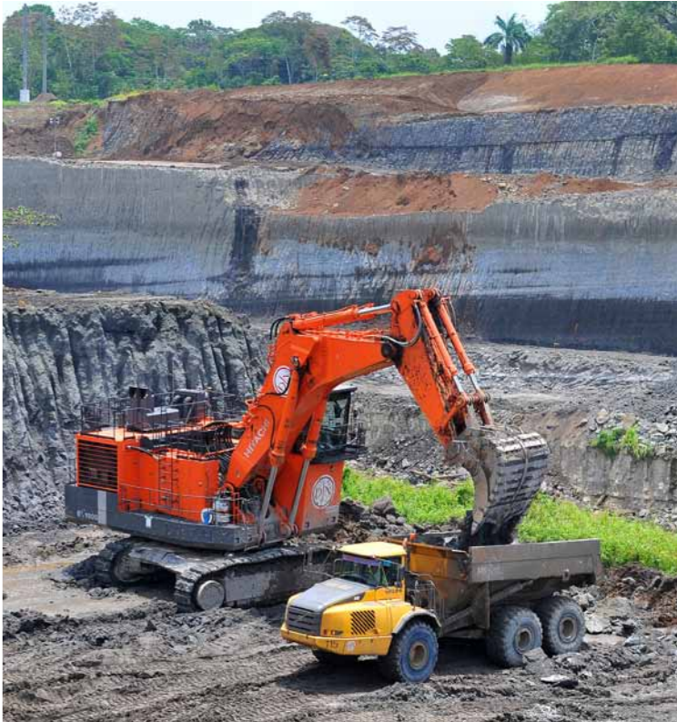
Excavation has been split into four contracts
