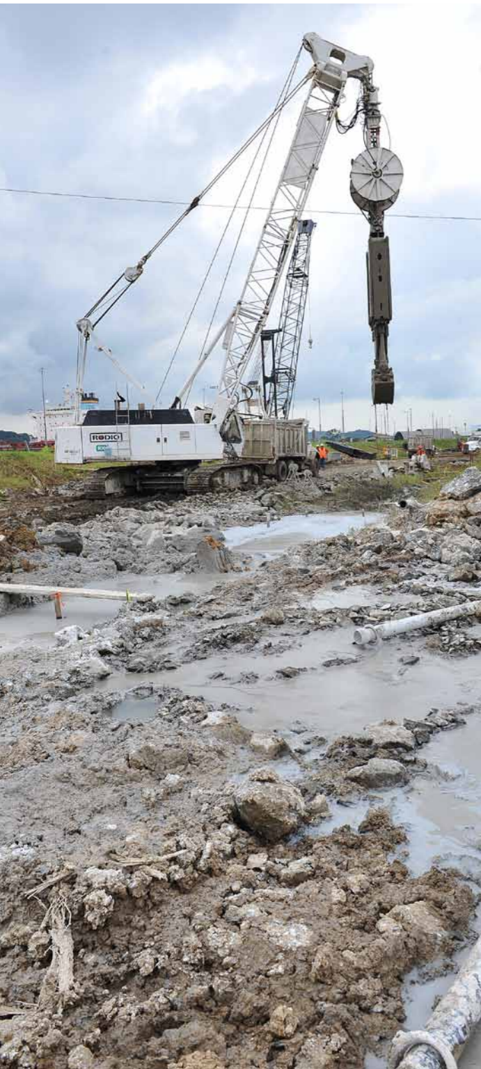
Construction of cement bentonite slurry wall between the northern end of the access channel to the new Pacific Lock and the exiting Pedro Miguel Locks
